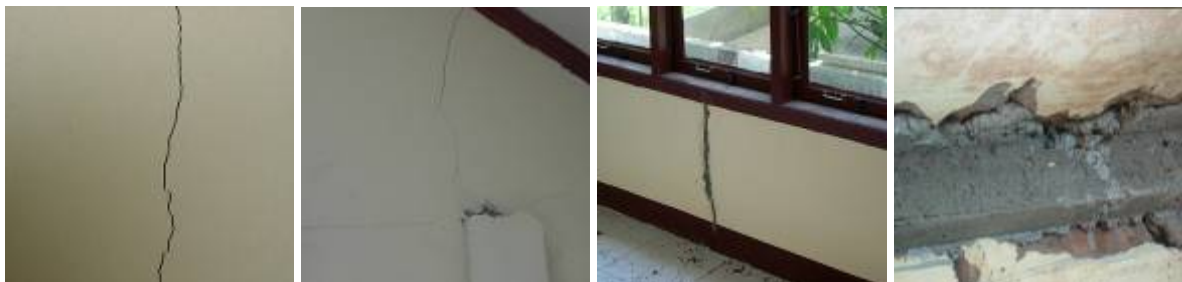
Figure 45 Existing Condition of SDN 13 Syamtalira Arun
