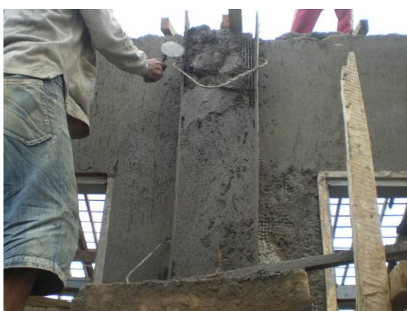
(a) Application of Iron Wire-mesh in Column Position
