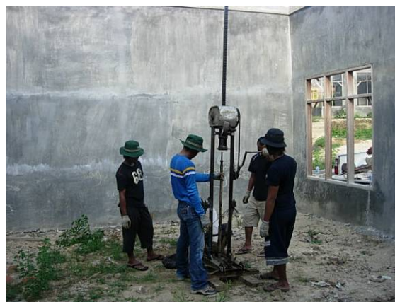
Figure 10 Soil Penetration Test
