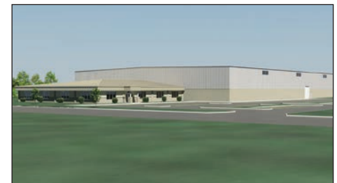
50,000-square-foot upgraded conventional facility
