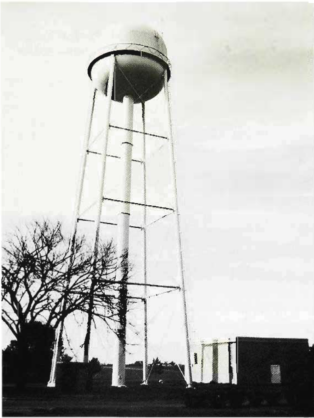
Double-Ellipsoidal Design. Dating from about 1950; Spreng's crew erected this tank at Willmar State Hospital in 1957.
