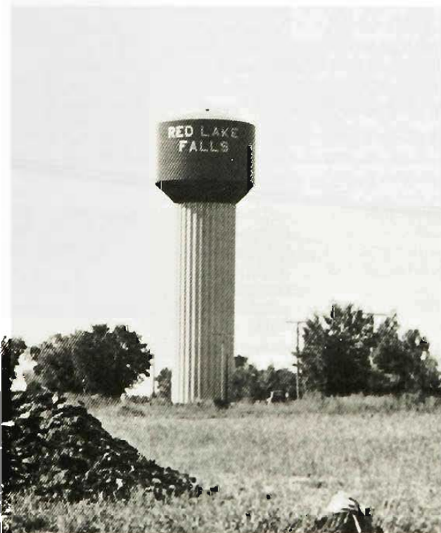
Hydropillar Design. Used from 1962 to the present; the author helped erect this Red Lake Falls tank.
