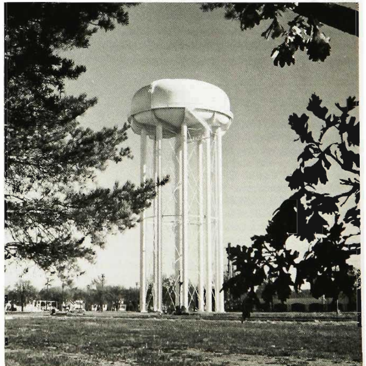
Torospherical Design. Popular from the 1950s to the present; Austin. Note central spiral staircase.
