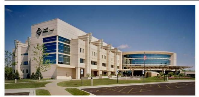
The expansion was restricted by the adjoining 70-year-old existing hospital and its relatively low 11'-2" floor to floor heights. In order to preserve interior space, the building utilities were aligned in exterior chases decongesting the ceiling plenum resulting in higher ceiling heights and a distinctive exterior aesthetic.
