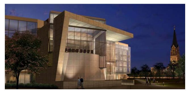
The diverse exterior of this research facility was composed of three cladding materials and four unique glazing systems. The result was meant to provide a signature building to the campus, expand the BioScience, Chemistry, and Physics departments, as well as introduce a Nanotechnology discipline to the university.
