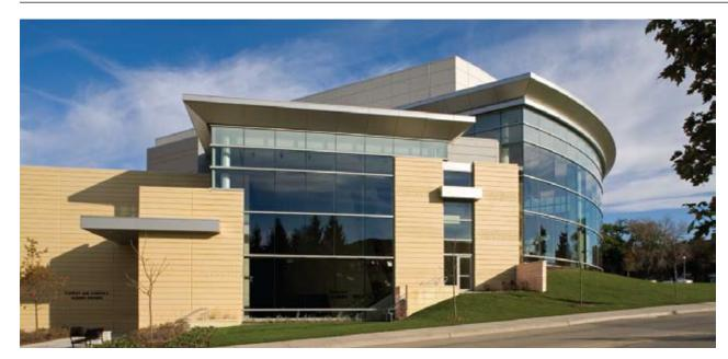
To meet the clients budget and schedule the building volumes were composed of exceptionally sized structural precast panels meeting the client's aesthetic expectations, rigorous acoustic considerations, seismic requirements and providing an iconic building for the campus.
