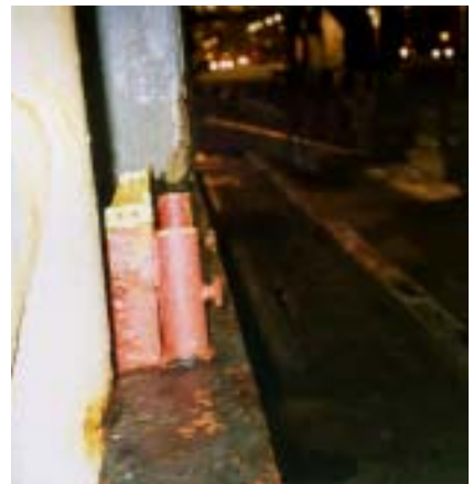
Sockets for removable handrails
