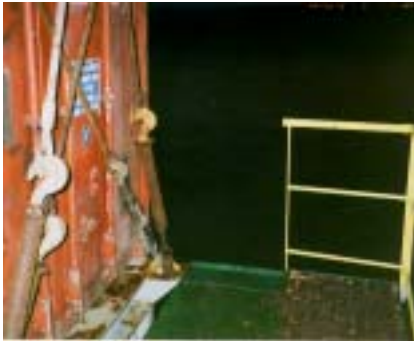
Typical gap in safety barrier
