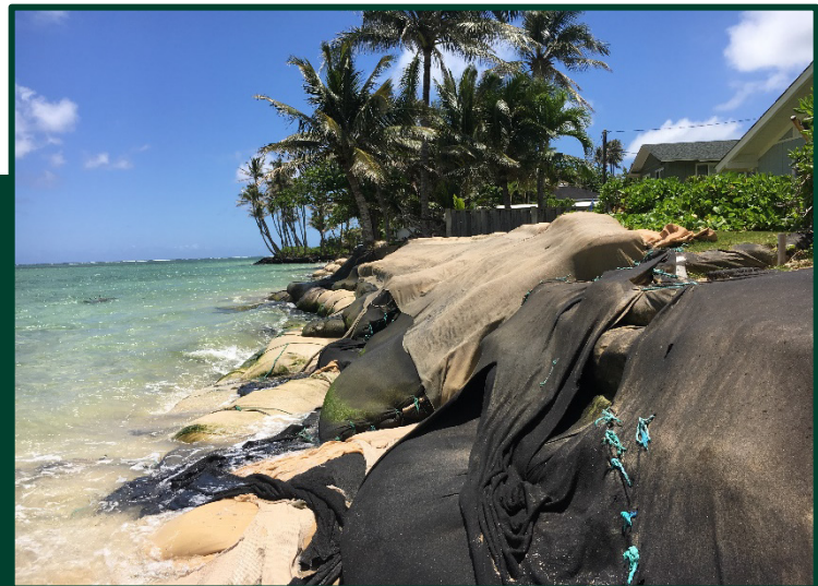
Figure 13. A truly resilient Hawai’i must employ nature-based solutions. When rooted in place-based value and knowledge, these solutions can be climate resilient, and are often less expensive and more effective than their conventional “gray” counterparts alone. Here, sandbags are used in a temporary attempt to protect property, and instead contribute to beach erosion. A living shoreline has shown to be more effective in protecting our beaches, and making a resilient coast. (Courtesy of Shellie Habel, DLNR-OCCL)
