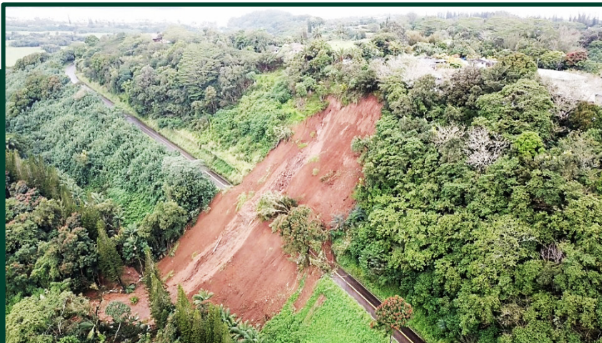
Figure 3. Heavy rainfall events and the resulting landslides and flooding have devastated areas throughout Hawai‘i, causing damages to homes, businesses, and transportation infrastructure. In March 2021, the islands of Maui, Kaua‘i (shown here), and O‘ahu experienced flashflood events that prompted the governor to declare a State of Emergency. As weather and rainfall patterns continue to shift, extreme weather events like these are likely to occur more often. (Courtesy of HIDOT)
