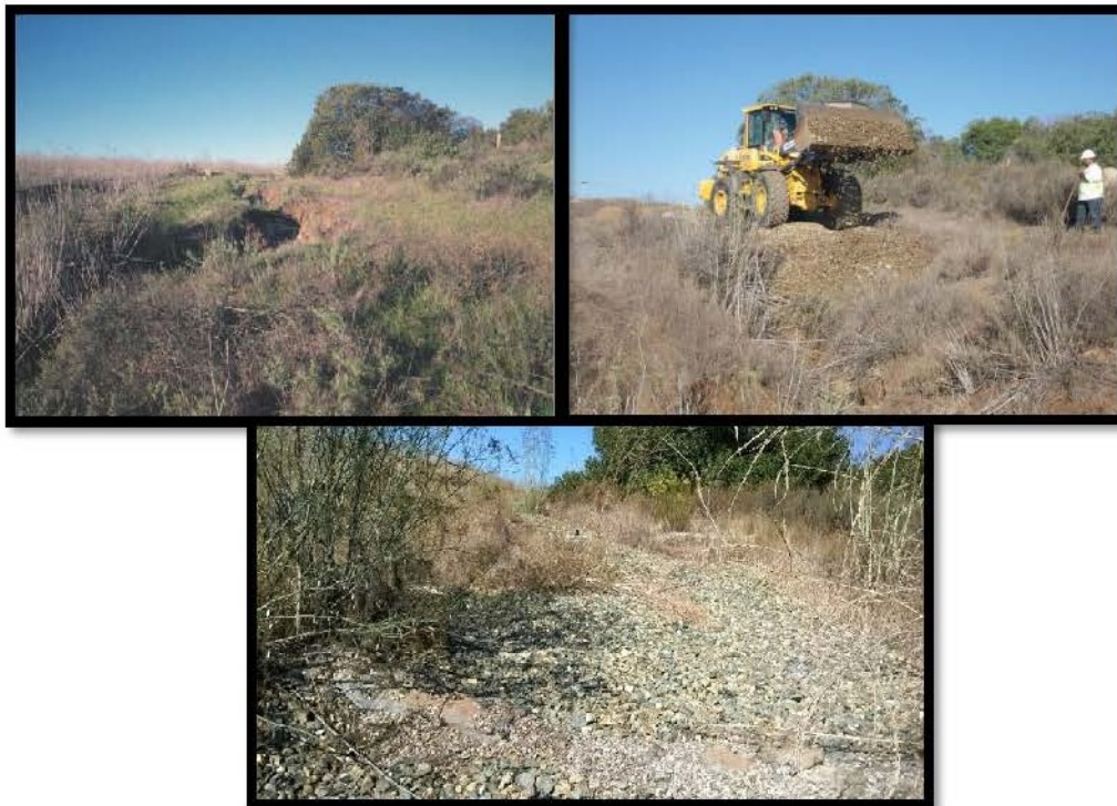
Figure 7. Area C: Deep Drainage Looking South, Crushed Rock Placement and After Treatment with 3" Crushed Rock and Check Dams.
