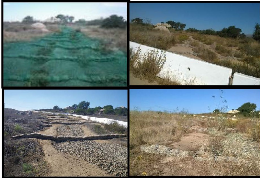
Figure 4. Area B1: Inside K rail, (Top Left) Check Dams and Hydro Seeding, (Top Right) After Treatment and B2 Outside K Rails, (Bottom Left) 3-Inch Crushed Rock and Check Dams, and (Bottom Right) After Treatment.
