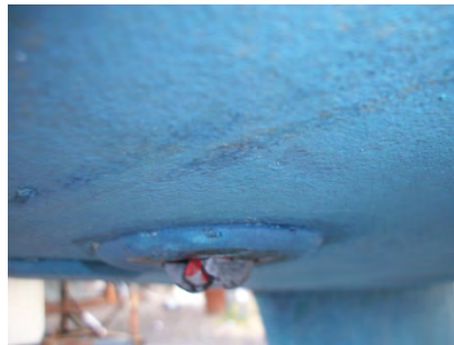
Fig 28 Log thru hull not tight to hull.
