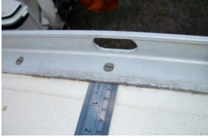
Fig 15 Slight area of lift stb side
