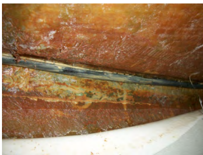
Fig 13 Hull deck bond from inside
