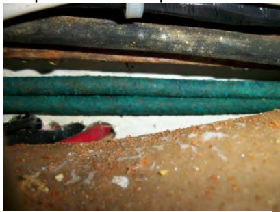
Fig 32 Fuel pipes in engine
