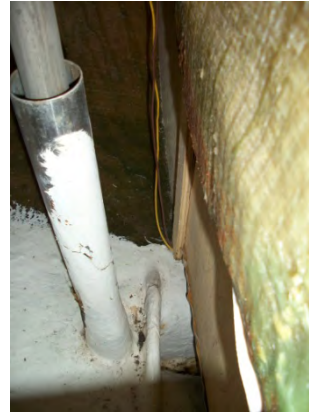
Fig 19a Rudder tube with open top above water line.
