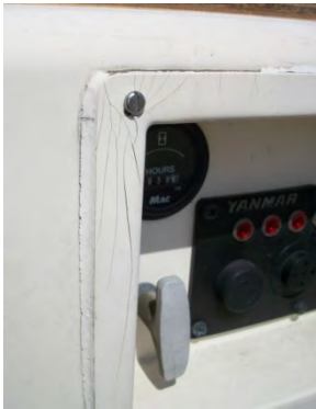
Fig 12 Crazing on engine panel moulding
