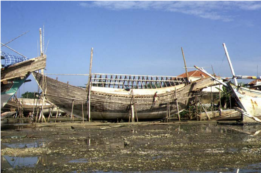
This janggolan under construction in 1994 was probably the largest ever built
