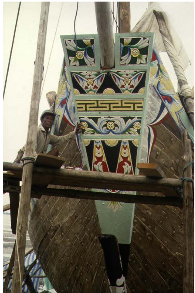
The bow of a timber-carrier janggolan under construction. The carved and painted decoration is traditional and had changed very little since the beginning of the 20th century.
