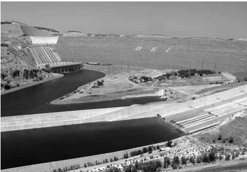
Figure 9.5. The Atatürk Dam on the Euphrates River in Turkey. Credit: https://www.flickr.com/photos/themua/ .
