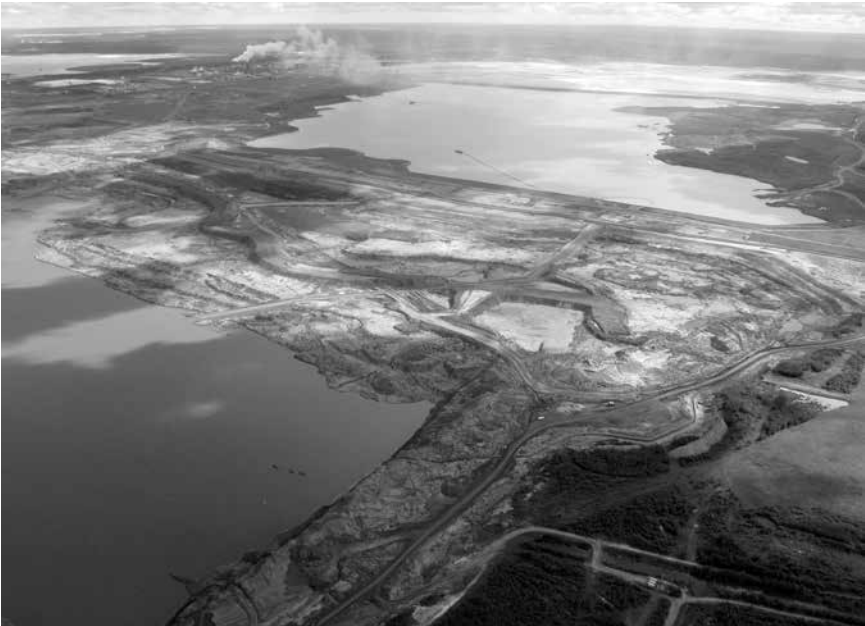
Figure 3.4. Tailings dam in Alberta—reputedly the largest man-made structure in the world. Credit: Jennifer Grant and the Pembina Institute. https://www.flickr.com/photos/pembina/7159711546/in/album-72157637876932305/ .
