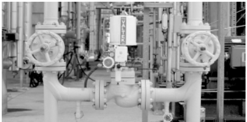
This 8-inch, back-pressure control valve operates in a liquid hydrocarbon plant with a 580 psi / 40 bar upstream pressure.
