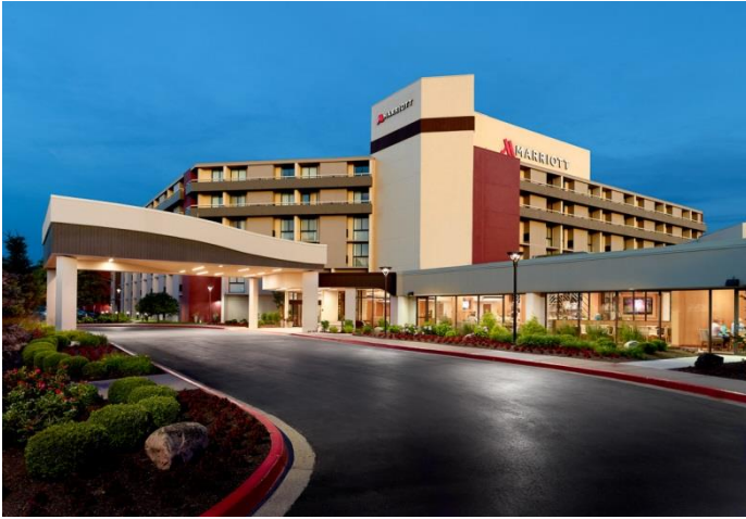
Hotel Main Entrance
