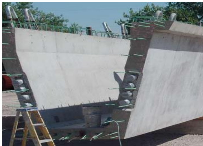
(b) Cross-section of U girders
