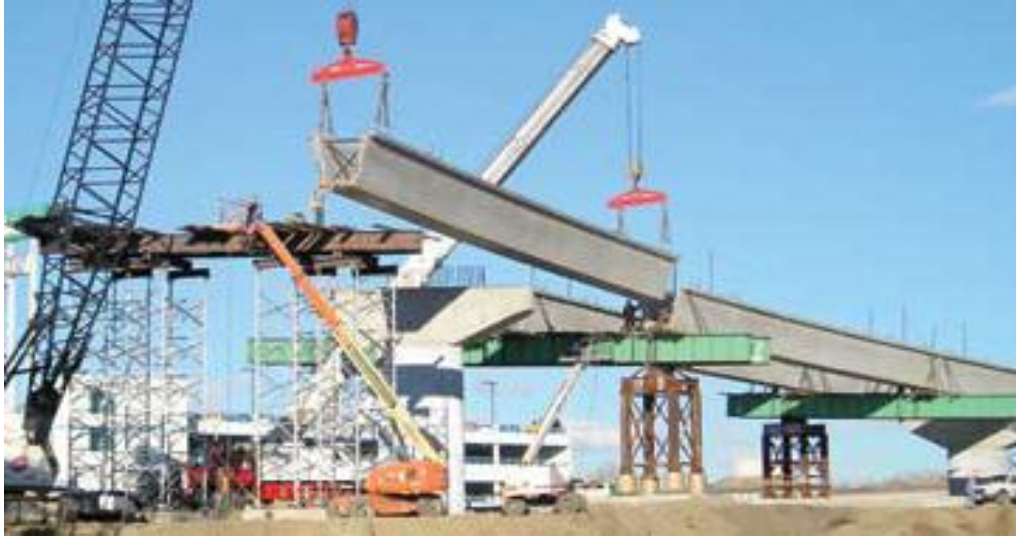
(a) Erection of U girders on site
