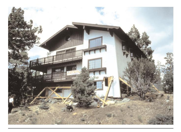
Here's a brand new beautiful house in Big Bear that suffered significant expensive, but unnecessary, damage in that earthquake. Unnecessary because the carpenters were unclear on the concept of a load path and installed the plywood only from the first floor up.
