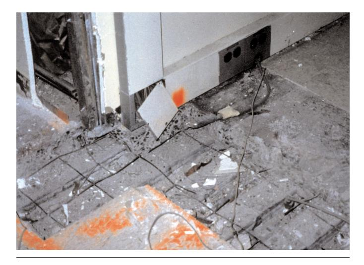
Upon investigation it turned out that the bars were never installed. There was no way to get the load to the walls at each end of the building. Ideally we need a system of checks and balances where if the contractor misses the placement of these bars the inspector catches it. Or even if the bars were missing on the shop drawings, the contractor should have asked why the engineer's plans and the rebar detailer's plans did not match.
