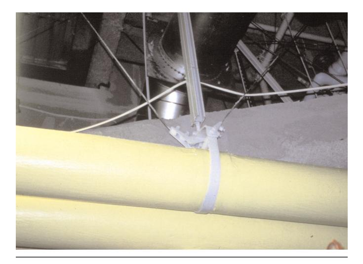
Here is a pipe where the longitudinal bracing is attached to only the hangar. The pipe can slide within the hanger because there is no direct connection between the bracing and the pipe. Unless the piping has flexible joint fittings, movement can cause breakage and leaking.
