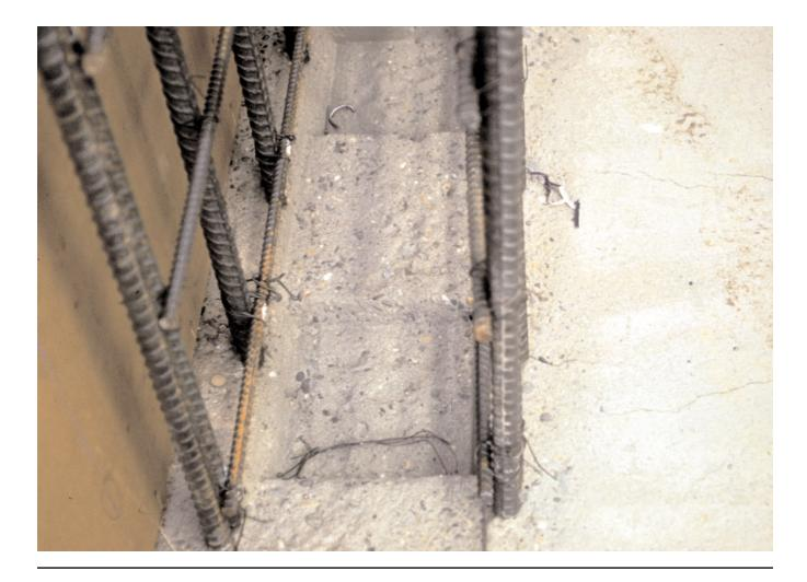
This is a horizontal construction joint in a wall. This is a very vulnerable element in a building. It is a weakened plane to begin with, and the joint is critical to the ultimate quality of the wall. Just before you pour the concrete you must make sure the joint is clean. Otherwise, during an earthquake, there will be a tendency for sliding along the joint.
