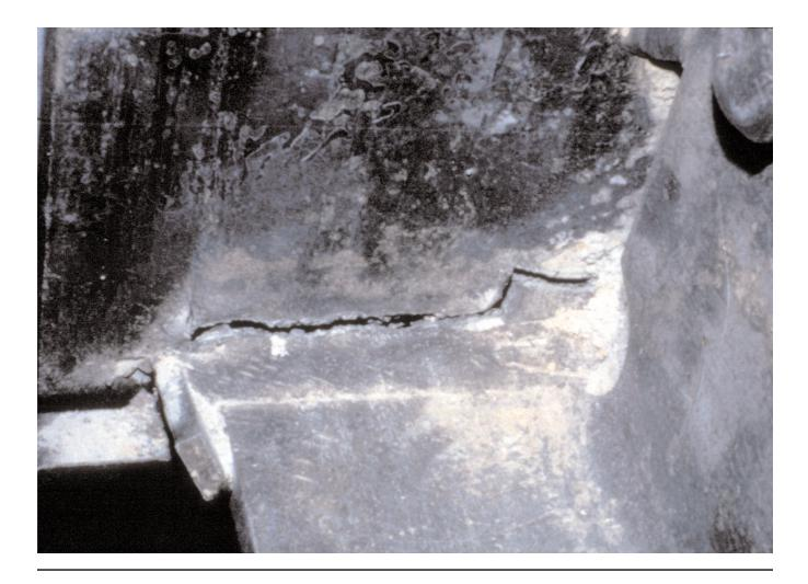
We learned in the Northridge, California earthquake in 1994 that without excellent quality control during the construction of welded moment steel frame buildings, we can end up with cracking in the connections. We need good quality inspectors overseeing good quality welders. Here we see a crack in the column where the bottom flange of a beam frames into the column. This connection is in a welded steel moment frame damaged in Northridge.
