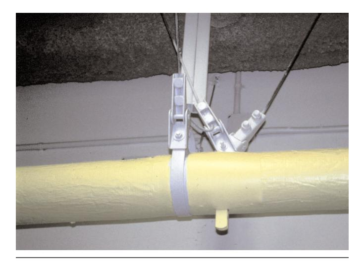
This slide shows wires providing longitudinal bracing for a pipe. The wires are connected to a ring clamp that is inside the insulation connected directly to the pipe, and should prevent longitudinal movement of the pipe.
