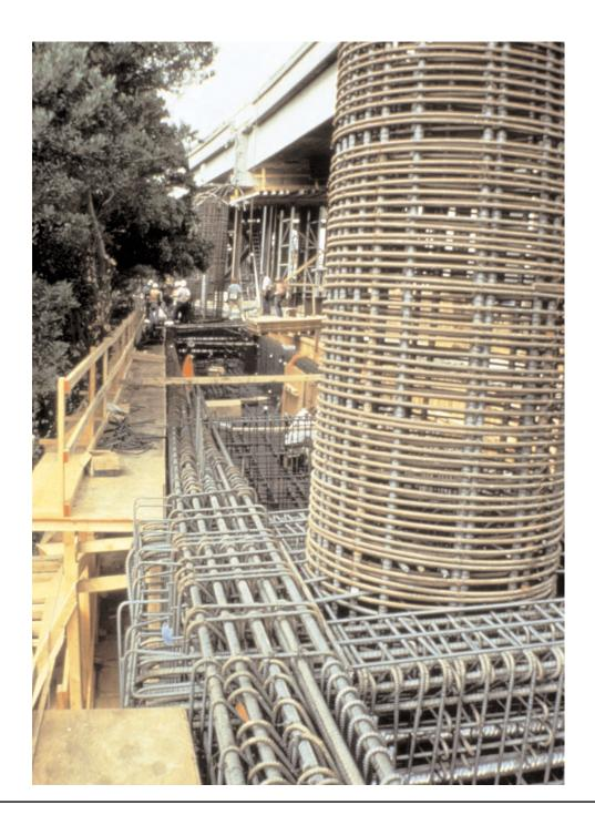
In earthquake country reinforcement is used to provide confinement for the concrete. Confinement is what gives concrete its ductility. Without proper confinement, concrete is brittle, and breaks apart under the movement caused by an earthquake.
