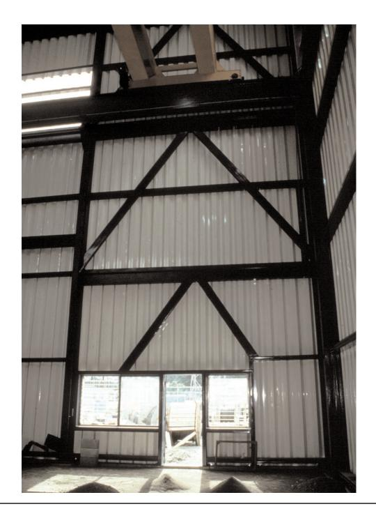
Quality control doesn't end with the construction of the building. It continues on with maintenance. This is a light steel braced frame building. After construction the windows were added, cutting off the braces. This modification completely obliterated the lateral system in this location.
