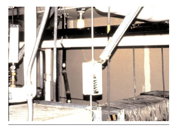
This box with the black spring in it is an isolator for a fan that is located in a duct. The isolator has a diagonal brace, which must have been intended for the fan itself. The isolator does not need bracing, but the in-line fan certainly does. Whoever installed and inspected the unit had no clue about the importance of bracing and its role in promoting proper performance in an earthquake.
