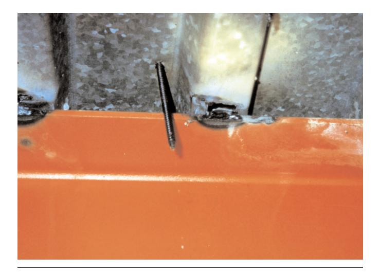
Unfortunately the welder welded right through the deck. There was poor quality control on the welder's part in making the connection, and poor control on the part of the inspector who didn't notice or didn't have time to check. Of all the deck to beam welds that were made, these are the most critical because it is at this location that horizontal earthquake forces are transferred to the frame that is designed to resist those forces.
