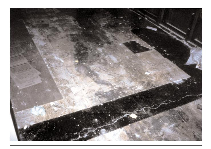
During the Loma Prieta earthquake a huge crack opened up in the floor diaphragm at the corner of the stair opening.
