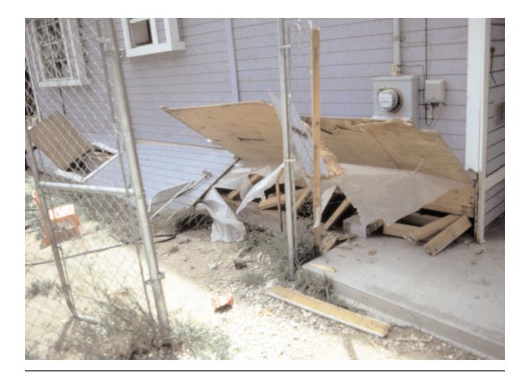
In this house, wood panels serve both as the structural sheathing and as siding. Carpenters had not properly nailed the wood siding panels on the cripple wall. So here, while the load path appears to be more complete than in the previous example, incomplete nailing of the edges of the siding resulted in this damage.
