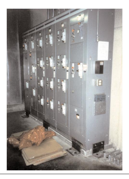
This is a motor control center in a hospital mechanical room. It is a narrow, top heavy piece of equipment. It is anchored at the bottom, but also needs to be anchored at the top so that it will not tip over. If it tips or shifts too much, the equipment it controls will fail, possibly making the building uninhabitable.
