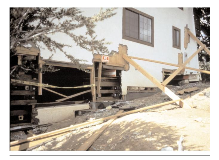
They put no plywood on the cripple wall between the foundation and the first floor. This critical portion of the house receives the earthquake loads from all the walls, floors, and roof. Earthquake forces exerted on a building accumulate in the lower portions of a structure, making the cripple wall construction critical. It receives the highest demand and must transfer the loads to the foundation. It was unable to do so in this case, due to the lack of plywood.
