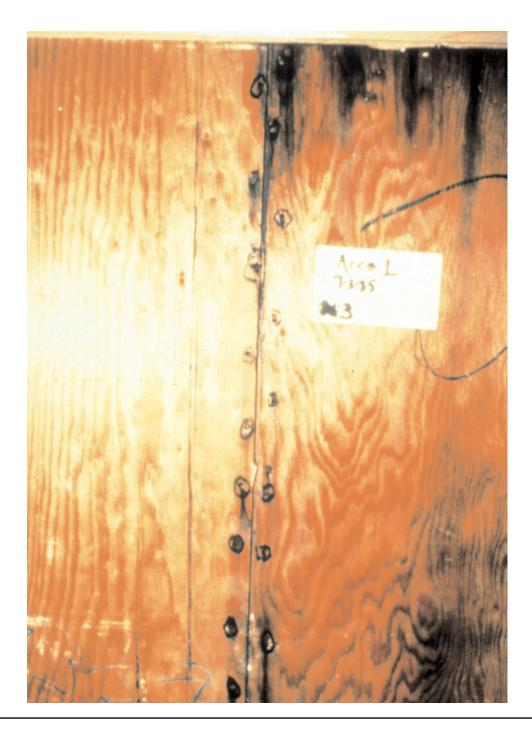
Plywood walls provide excellent earthquake resistance in earthquakes if they are installed properly. In order for a plywood wall to be effective, it relies on nails. These nails must be of the proper size, spacing, and with the proper edge distance. They cannot be overdriven, or the plywood will lose its strength.
