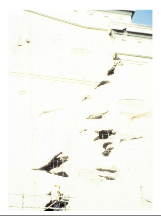
They took out a lot of loose material. Without appropriate vibration to consolidate the concrete as it is poured, and close observation by inspectors during concrete pouring operations you can get rock pockets and voids which seriously weaken the walls.
