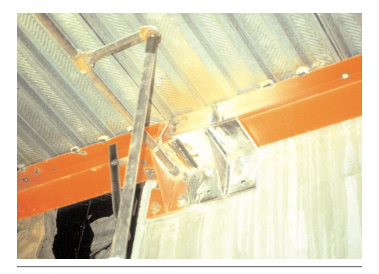
This is the inside of a two-story steel braced frame in Palo Alto, California damaged in the 1989 Loma Prieta earthquake. Problems were caused in that earthquake because the roof diaphragm has to be able to transfer the load to the steel braced frame. As you can see here the roof deck was a steel metal deck without concrete fill. This deck acts as a diaphragm and the load should have been transferred through a direct connection between the deck and the frame.
