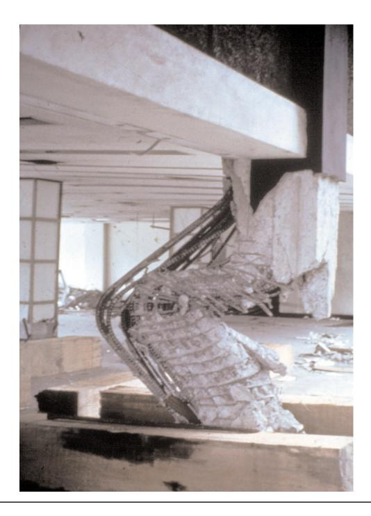
This is a concrete column that supported a 5-story concrete office building that was damaged in the 1972 Philippines earthquake.
