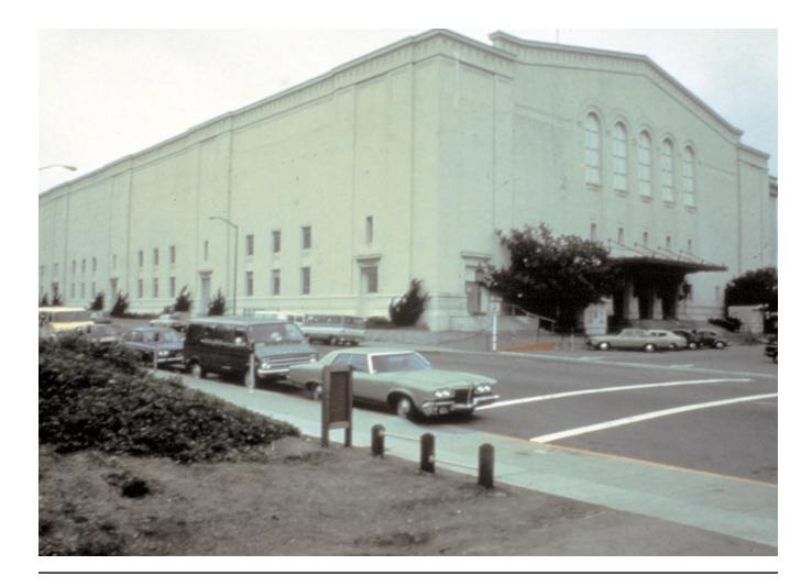
This is the Kaiser Convention Center in Oakland, California. During an evaluation of the expected seismic performance of the building, conducted as part of a renovation, concern was expressed about the quality of the concrete in the walls. The engineers listened, by tapping along the walls at various intervals and decided that the walls sounded hollow.
