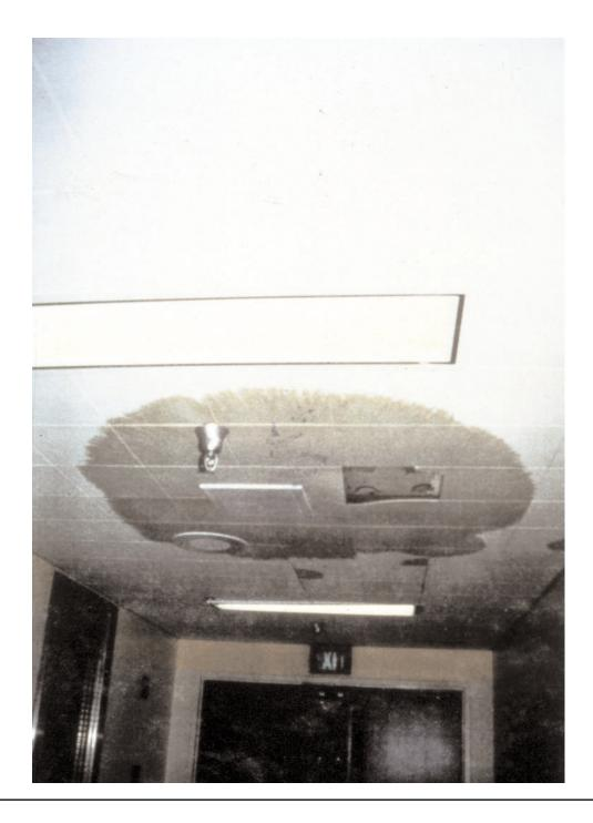
There were many leaks caused by breaks of the reheat coils—to limit the release of water they need flexible couplings where the waterlines connect. Imagine what happens to the furnishings and equipment below this leak.
