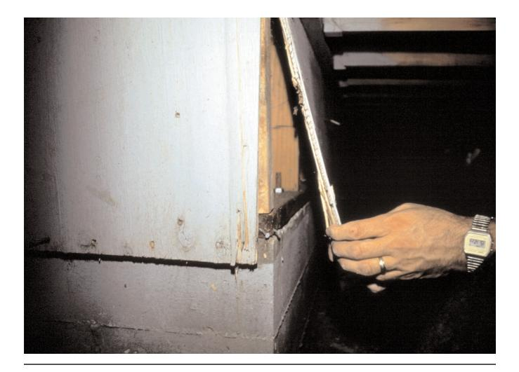
In Big Bear, California, after the 1992 earthquake there, we saw tremendous damage in modern wood frame construction, caused by construction and inspection errors. Here we can see damage caused by nails that were overdriven or placed wrong. In addition, the vertical edge nails were missing. The plywood just peeled off, unable to transfer the load.
