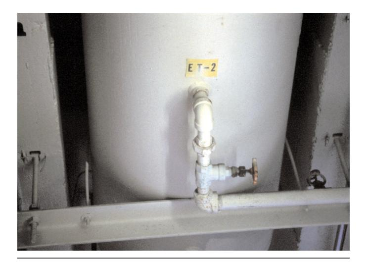
Here we see an overhead tank on a trapeze suspended from the structure above. The piping coming out of the tank feeds a piece of equipment below. Neither the tank nor its trapeze is braced, so in an earthquake it will swing. This motion will cause the piping or its connectors to break. In this case, the installer and inspector both should have known better.
