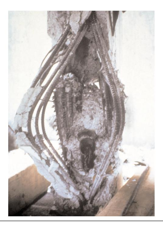
The column failed because all of the column ties were cut so a roof drain could be installed. This is what happens if you have no ductility. This is a dramatic illustration of the effect the "non-structural" trades can have on a building's performance in an earth-quake.
