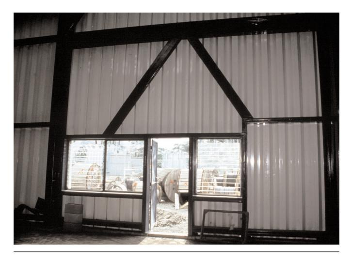
The bottom braces won't do any good in an earthquake because they are unable to transfer any kind of earthquake load from the frame above to the foundation.
