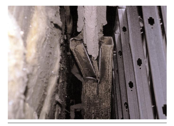
Dozens of steel braces failed in this building. One reason is because of incomplete welding of the brace to the gusset plate. The right side was welded and the left side was not.
