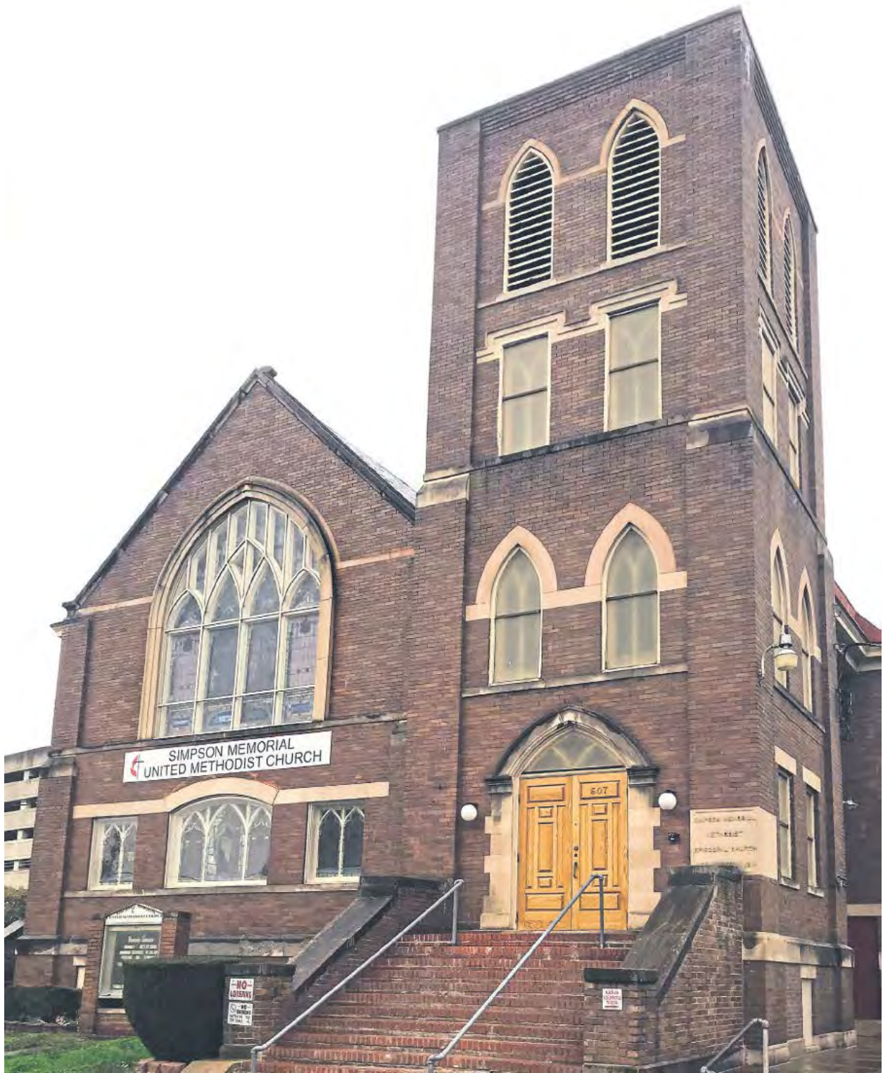
Simpson Memorial United Methodist Church on 607 Shrewsbury St. was formerly known as the Simpson Memorial Methodist Episcopal Church. The structure was built in 1914 and served as an anchor of Charleston's African-American community. By Stan Bumgardner For Daily Mail WV
