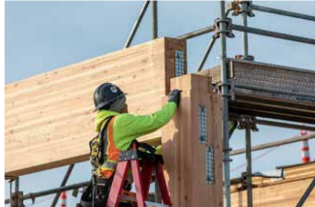
Installation of beam using concealed pre-engineered beam connectors
