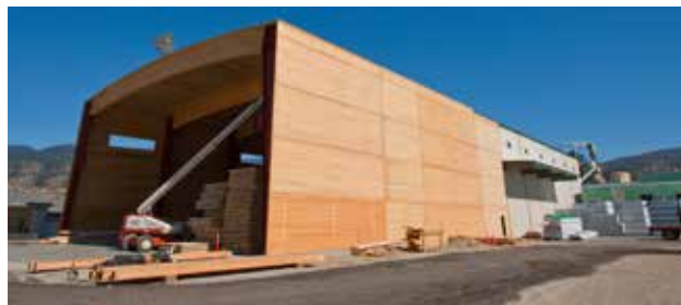
Structurlam Mass Timber Corporation Factory Addition, Okanagan Falls, BC, Canada
