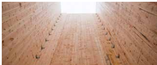
Elevator Core Shaft
