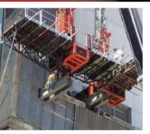
protection systems, while its Hydro Mobile division manufactures four series of mastclimbers, each with specific users and applications in mind. The M-Series mastclimbers - billed as the company's workhorse - are aimed at high capacity masonry, demolition and heavy block and stonework and are a ratchet driven, broad platformed product particularly suited to heavy
