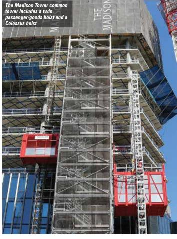
Balfour Beatty's façade manager on the project Jack Bird says: "The Madison project has two large programme critical components - the bathroom pods and the curtain wall stillages - both of which must be transported vertically and distributed to the floor plate by the Colossus hoist which has been specifically sized to ensure the largest pods - measuring 2.7 by 2.8 by 2.55 metres - can be delivered safely to site."
