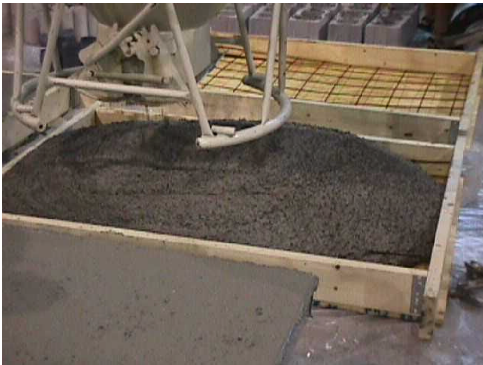
Figure A.1. Placing Concrete in Wood Forms.
