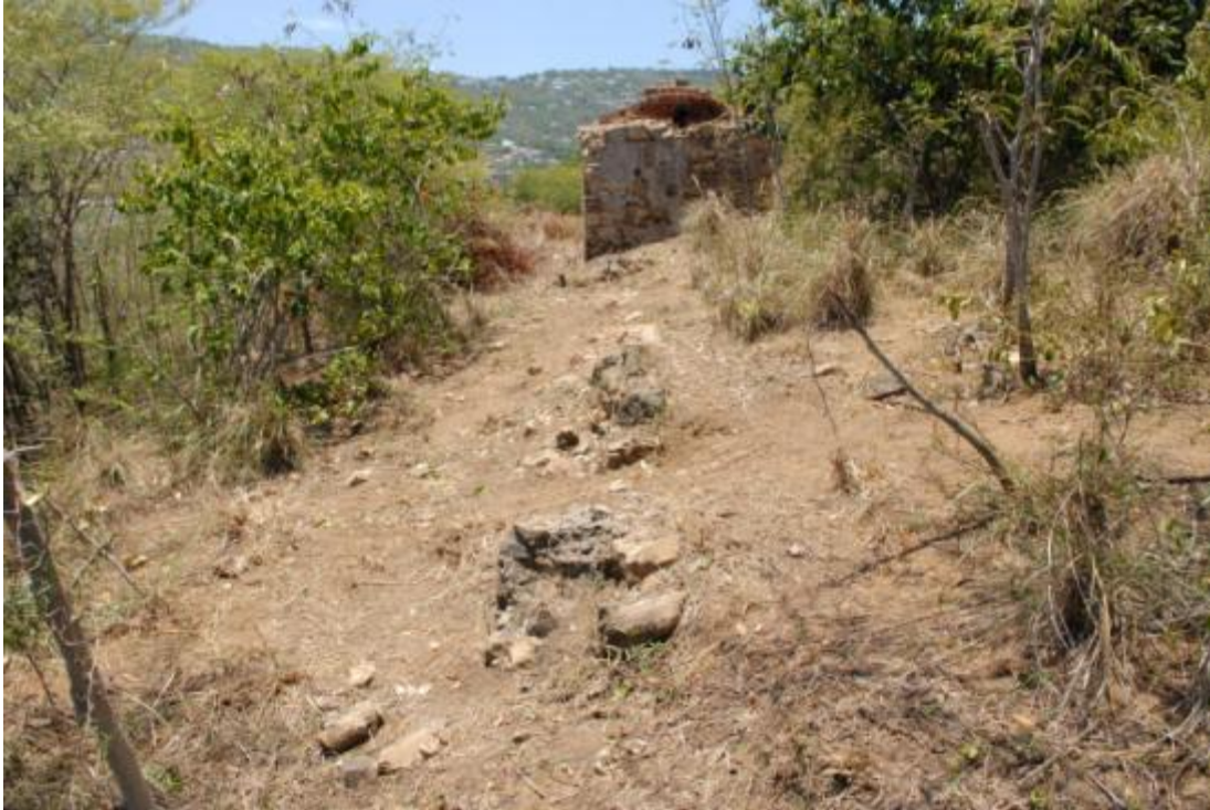
Figure 5-9. Foundation C, facing north towards the cistern. Photo taken in 2008 by the author.
