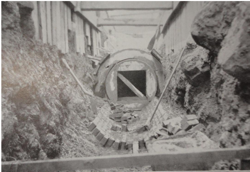
West End Main Drainage System, showing Hinton Avenue Section, August 15.
