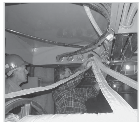
Installing MaxCell
