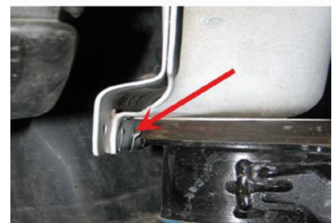
Inspect the washer-to-cradle clearance and the cradle-to-frame rail flange clearance.
