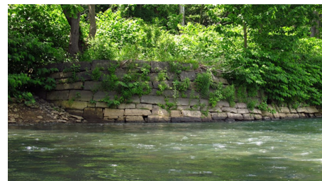
Canal Wall - Packsaddle Gap (Courtesy of Mike Mance)
