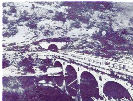
Canal Conemaugh Aqueduct
