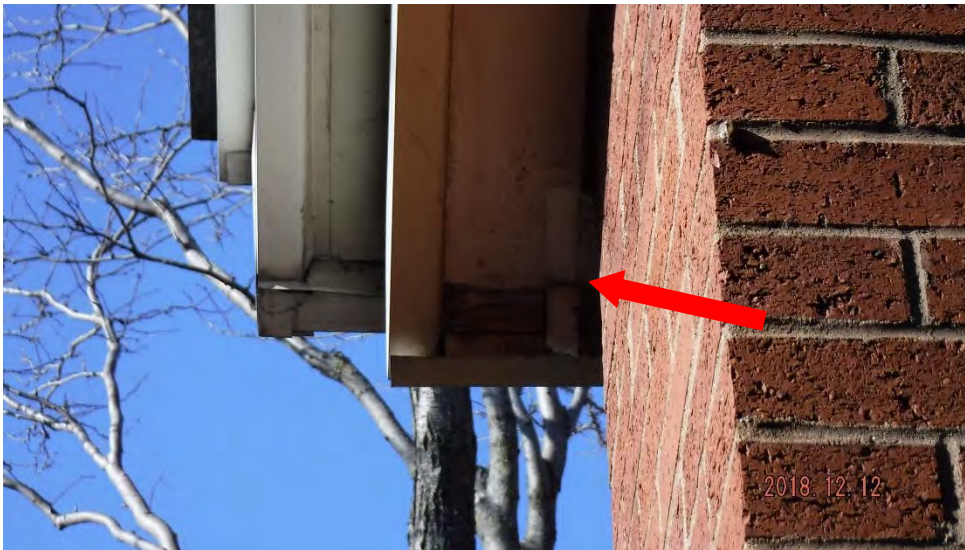
3c. Disrepair of soffit and chipping/flaking paint (see #3 on elevation photo for typical location).
