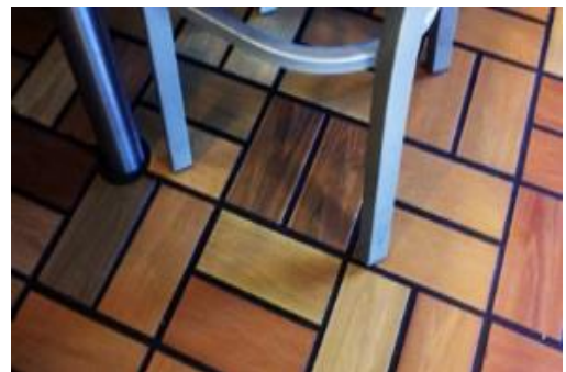
Floors after being cleaned properly
