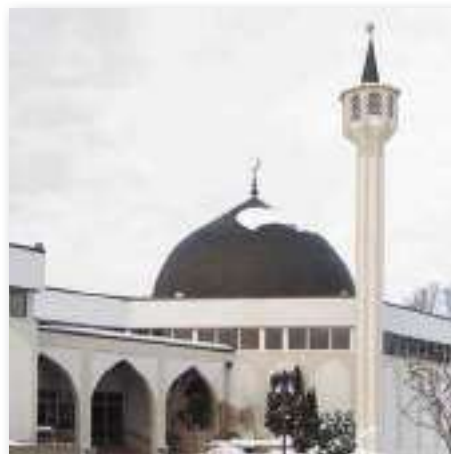
Canadian Islamic Centre (Al-Rashid), Edmonton, Alberta
