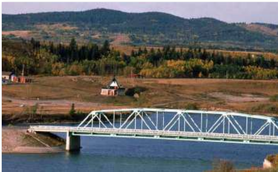
Truss bridge over the Bow River in Morley, Alberta located on Chiniki First Nation territory.
