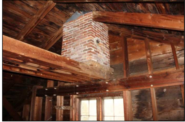
Center left: (58) Attic roof framing with ladder to belfry; Center right: (59) Attic detail of chimney remnant supported on beams (south end)
