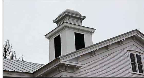
Two rows above (clockwise from upper left): (9) Detail of front pediment; (10) detail of front entry and doors; (11) Detail of cupola/belfry and gable raking cornice; (12) Detail of northern chimney on standing seam roof
