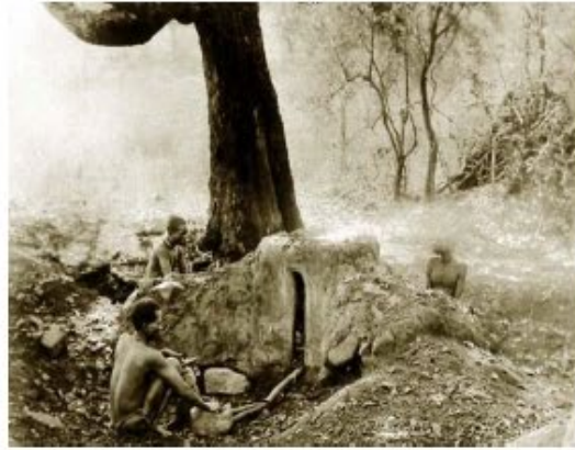
Venda-type iron smelting furnace from 1888
