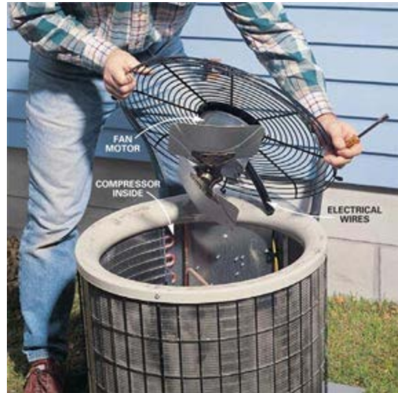
Figure C-3. Removing of the top of the condensing unit for cleaning (Source: thefamilyhandyman.com, reprinted with permission).
