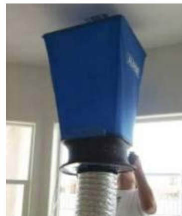
Figure 8. A powered flow hood in use.
