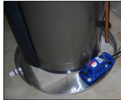
Figure 11. Proper HPWH installation
