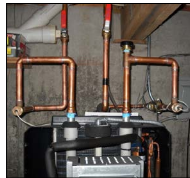
Figure 13. HPWH with heat traps
