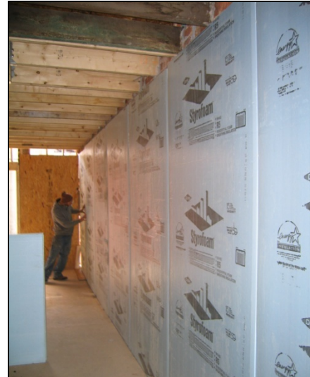
Figure 5. XPS used by Chesapeake Habitat for Humanity
