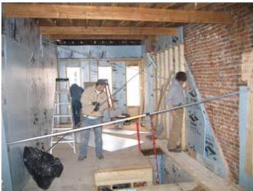
Figure 11. Bracing insulation on opposite walls
