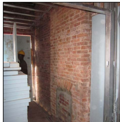
Figure 9. Example of wall ready for insulation
