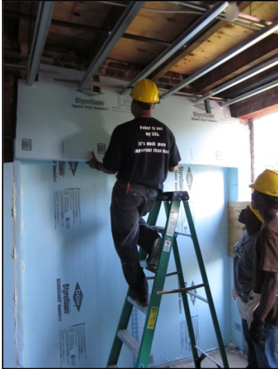
Figure 16. Install insulation from below
