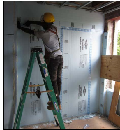
Figure 13. Tape over seams less than 1/8" wide
