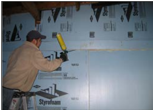
Figure 14. Use foam to seal all seams greater than 1/8" wide
