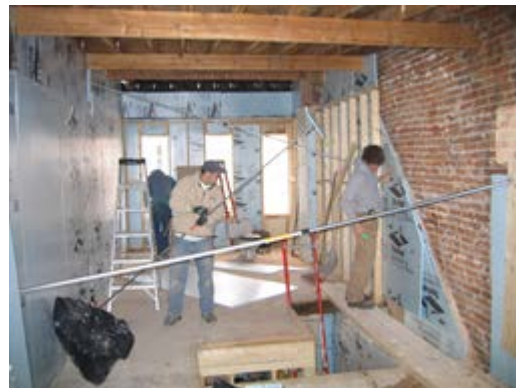
Bracing opposite sides with extension poles
