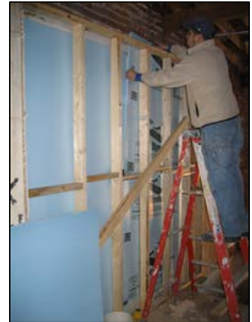
Figure 21. Slide insulation in behind existing stud wall
