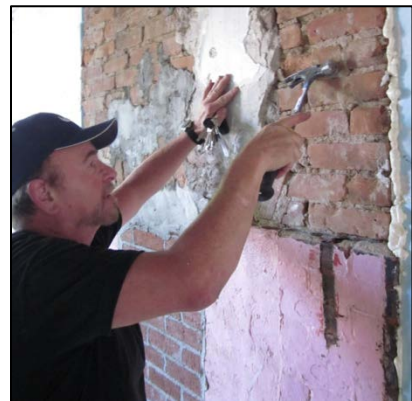
Figure 8. Knock off all debris, nails and plaster from wall
