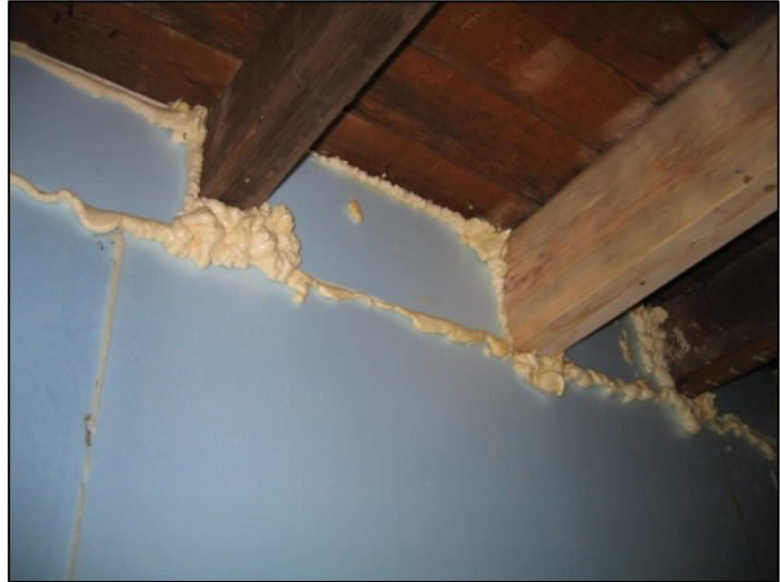
Figure 17. Seal all seams with low-expanding foam
