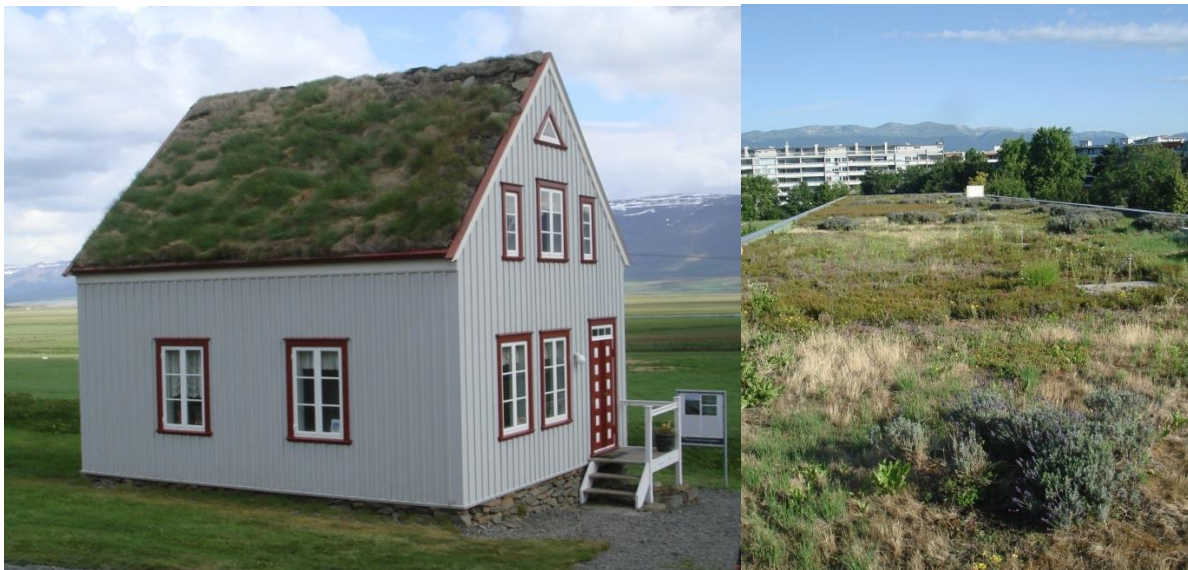
Figure 3.6: Green roofs: House in Iceland and flat roof in Geneva.
