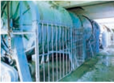
■ RAW MATERIAL MILLING AND MIXING
