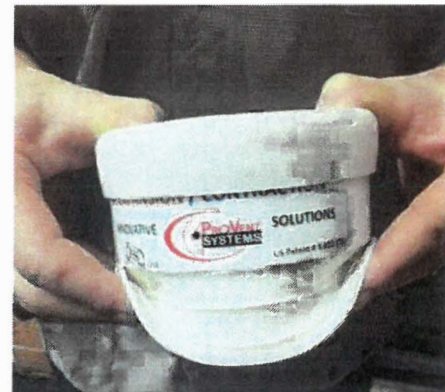
Roll both flex ends to meet each other
