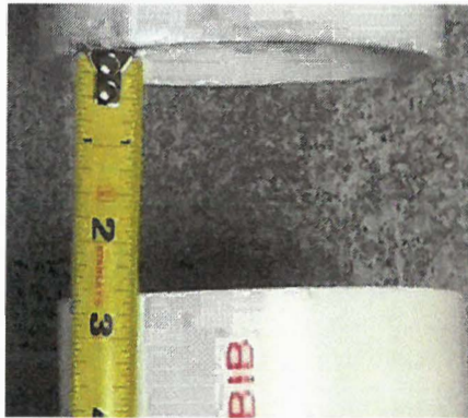
Insert a 2-1/2" gap between the pipes
