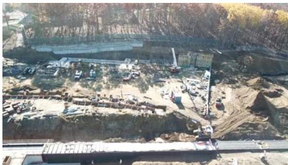
Aerial View of Foundation @ Science 1
