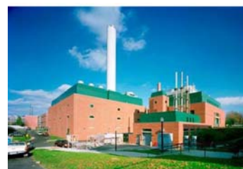
Central Utility Plant
