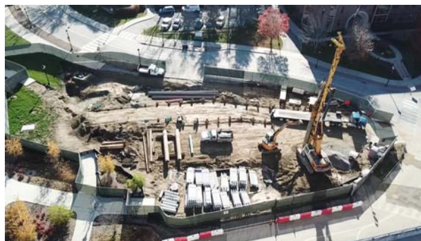
Aerial View of Tunnel @ North Garage
