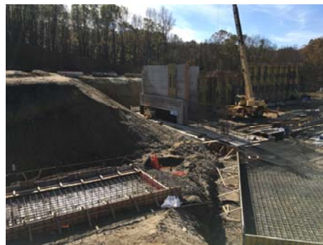
Foundation @ SUP & Utility Tunnel
