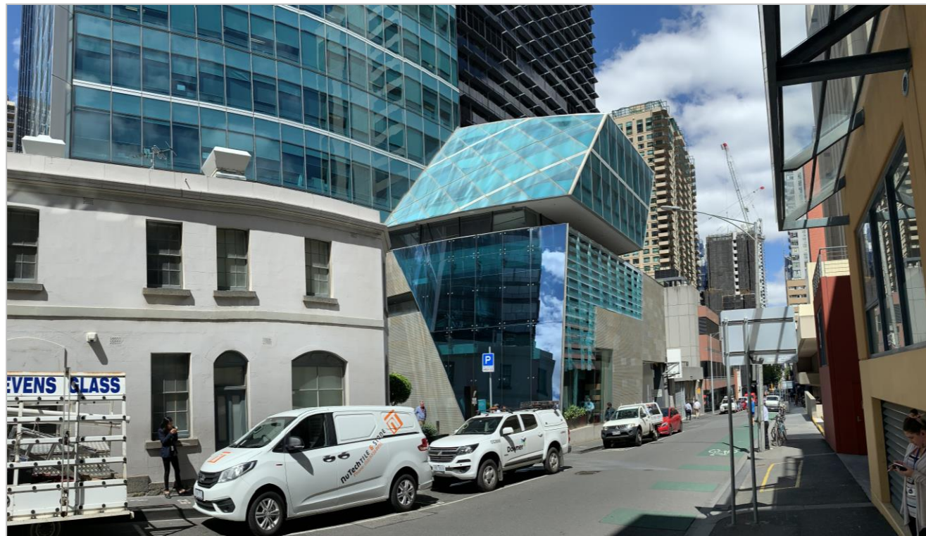
Figure B3 – 50 Lonsdale Street – The Urban Workshop
