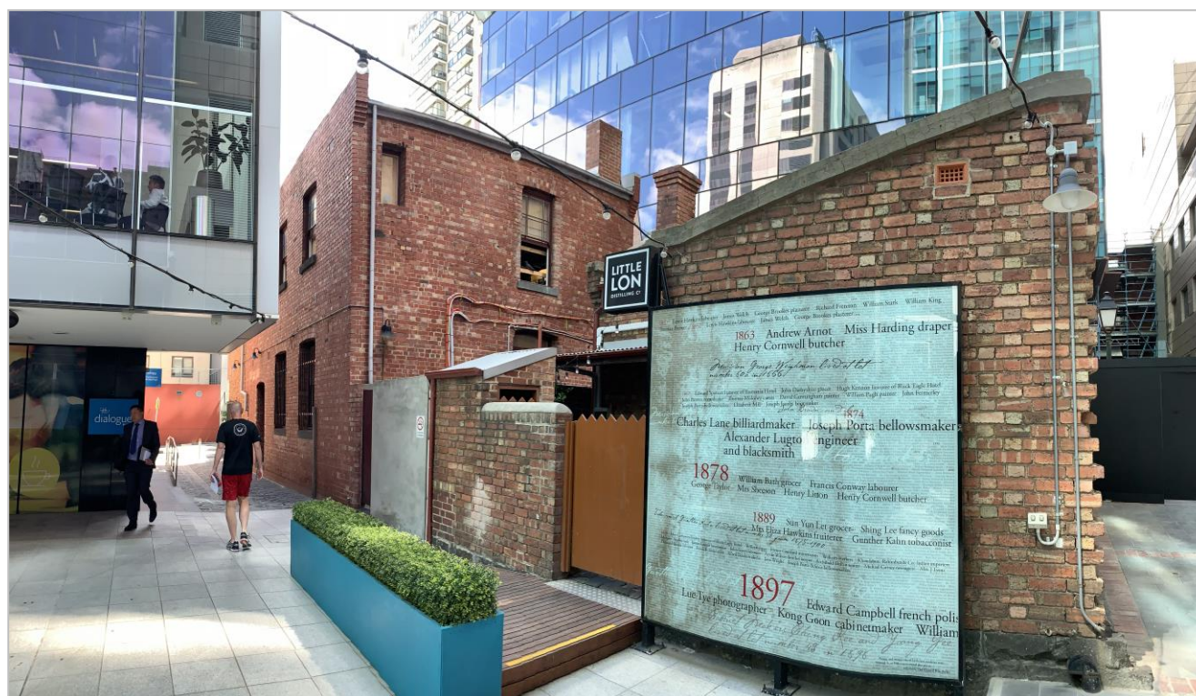
Figure B5 – 50 Lonsdale Street – The Urban Workshop
