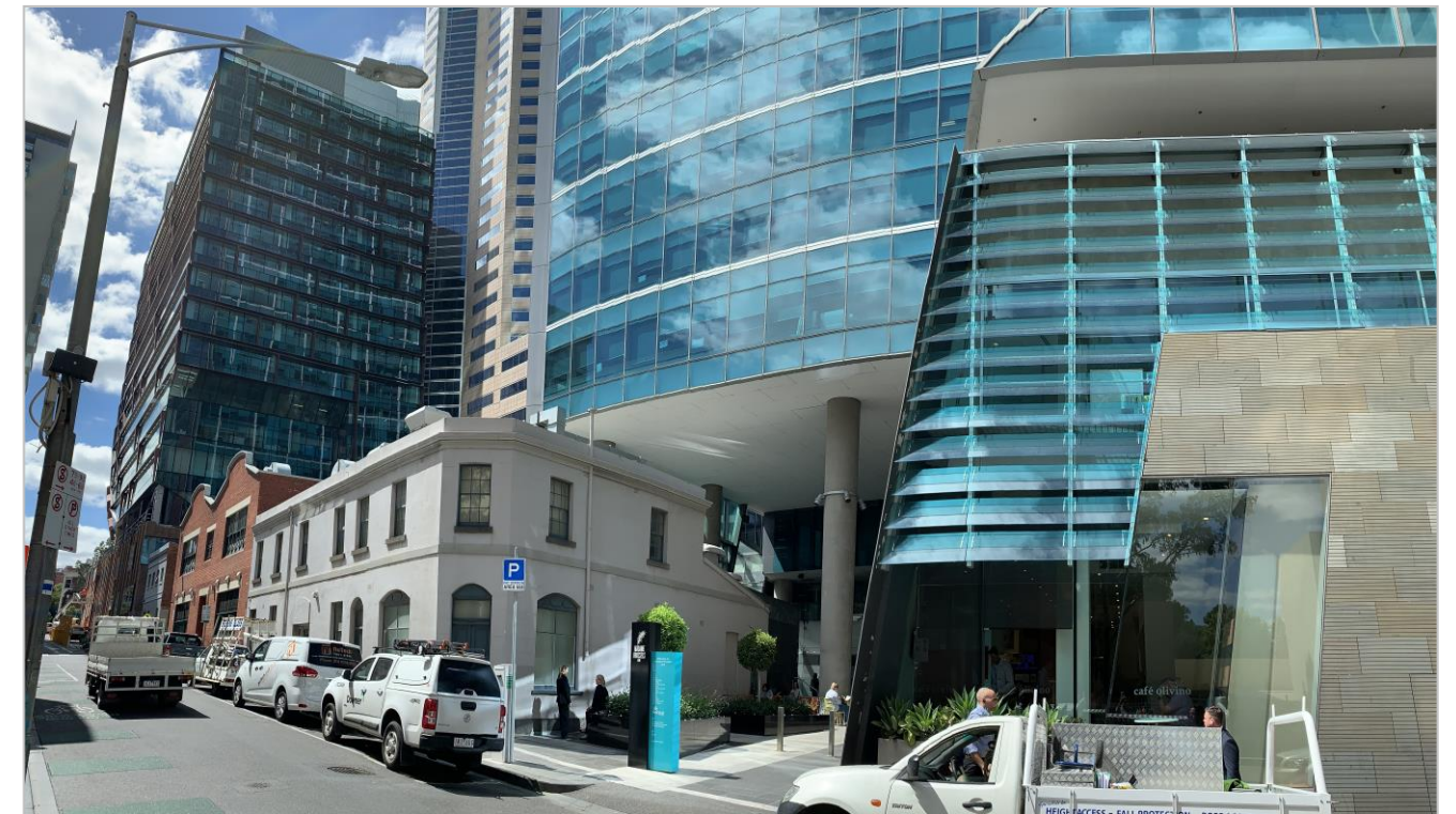
Figure B4 – 50 Lonsdale Street – The Urban Workshop
