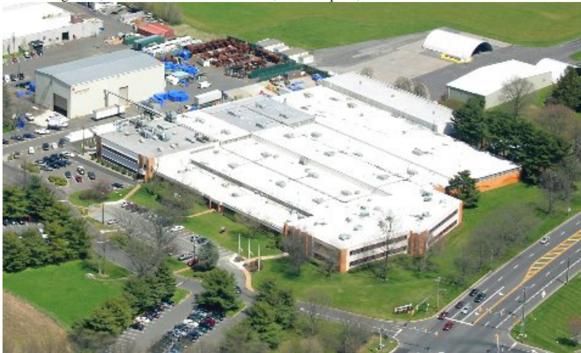
Arial view of Inductotherm Corp.
