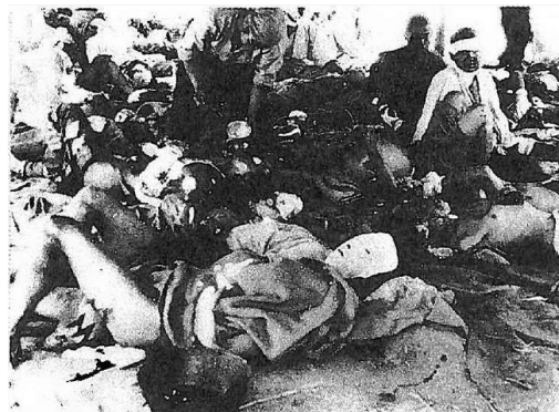
Aid station in chaos (Red Cross hospital), August 10, 1945
