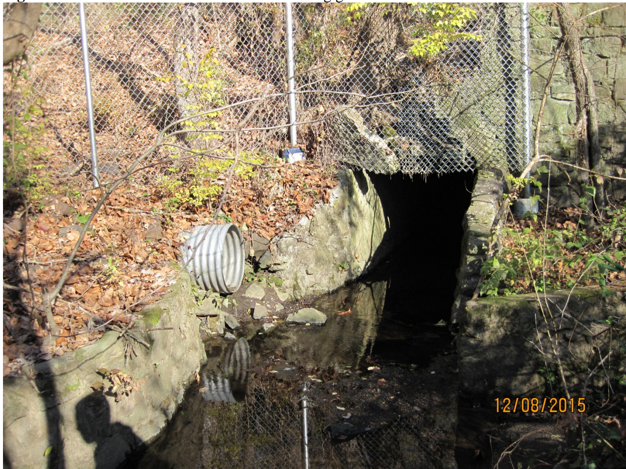
Figure 7: Stone culvert to be closed off with swing gate.
