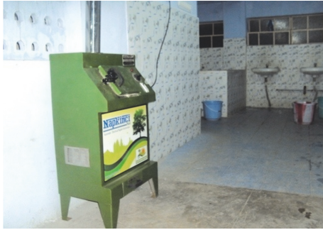
FIGURE 3: Incinerator installed in the toilet for easy sanitary products disposal. Source: http://www.vendingbiz.in/sanitary-napkin-incinerators-napkinci-maxi-1902444.html .
