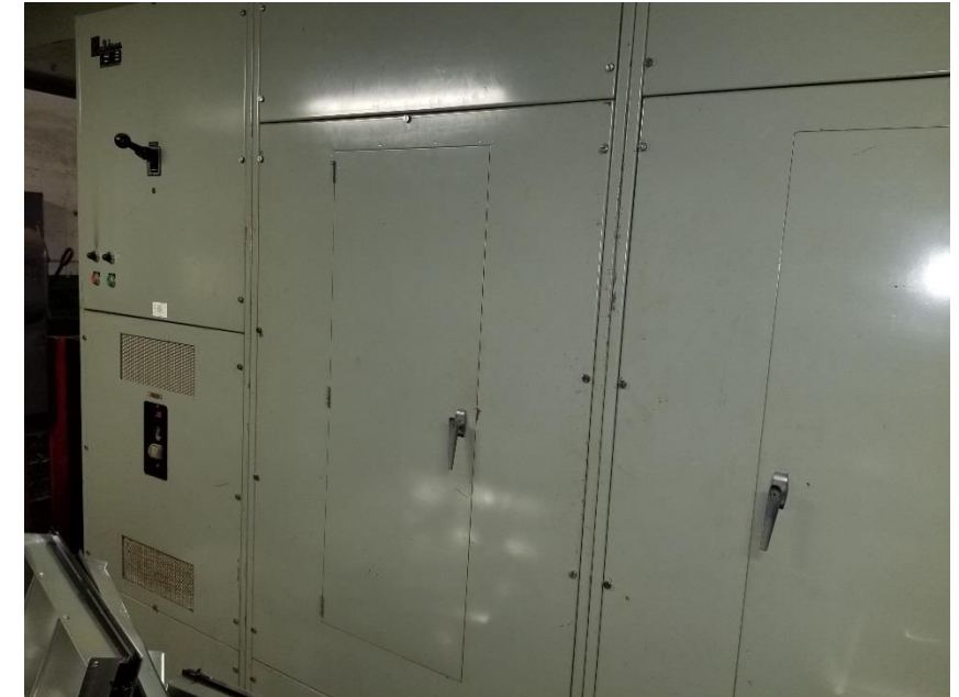
Live-front Distribution Equipment – Basement Electrical Room
