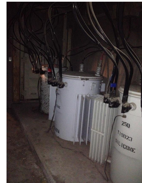
Indoor Transformers Feeding First Floor Electrical Rooms
