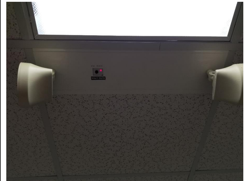
Emergency Lighting – Ceiling Mounted
