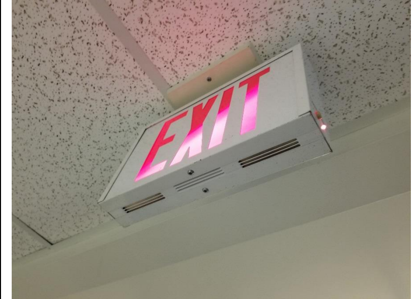
Emergency Lighting – Ceiling Mounted
