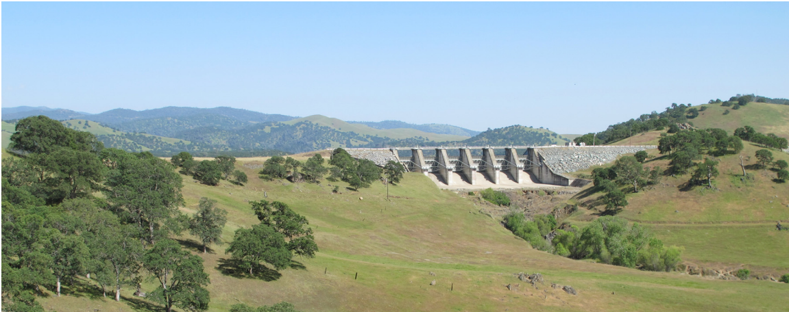
Gated service spillway at right. Emergency spillway is flat gap on the crest of hill to the left.
