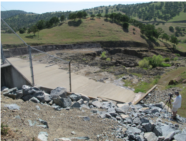
2012 view of Exchequer gated spillway apron
