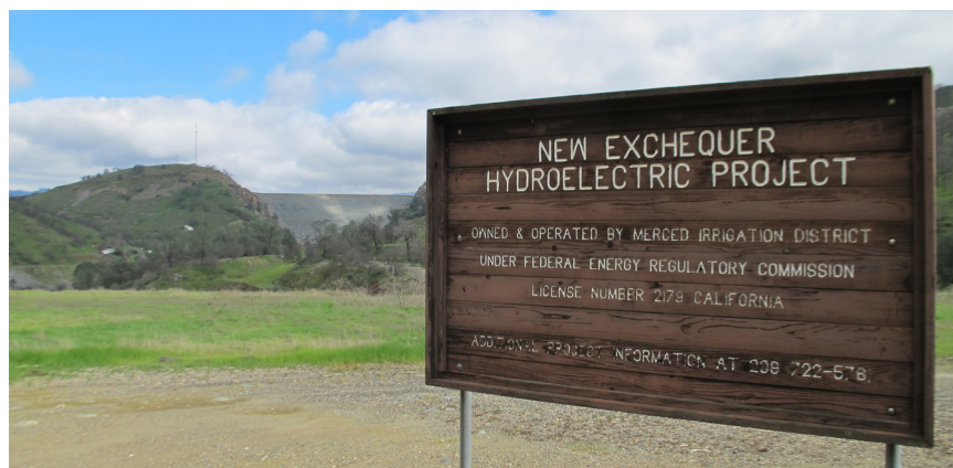
The Exchequer main dam is in the distance to the left of sign. Powerhouse and river outlet are at base of dam out of view. Spillways to the left out of frame.
