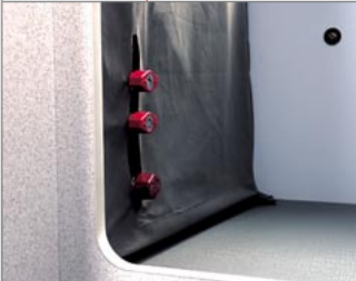
Gasabsperrventile
