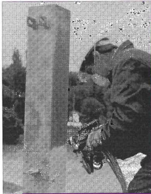
Fixtures such as bridge railings that cannot be removed for galvanizing can be sprayed with Zinc or Zinc/Aluminum for corrosion protection.
