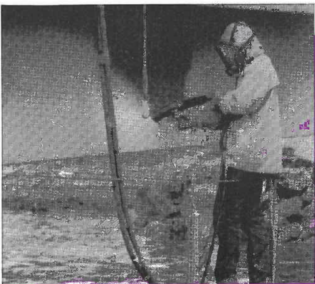
The operator can control the coating thickness in one application. Zinc metallized coatings are dry on contact.
