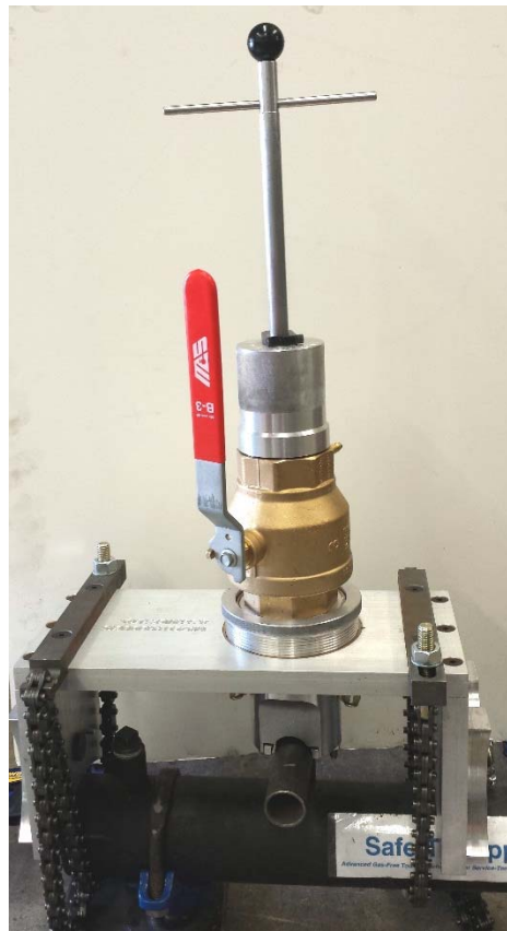
Platform is secured over tee.
