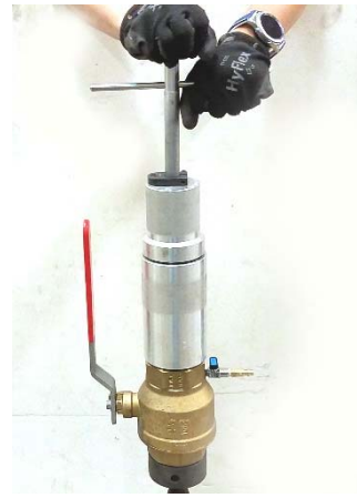
Remove punch, then insert Self Tapping Plug into main
