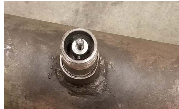
Rubber plug shown in nipple.
