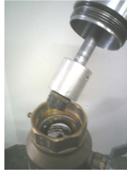
Plug removed. Held captive by the magnet.
