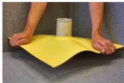
3) Fit and adhere the membrane piece properly around the pipe into the fresh applied adhesive. Make sure that the membrane upstand (3/8") fit and is adhered and pressed properly with sufficient adhesive below.
