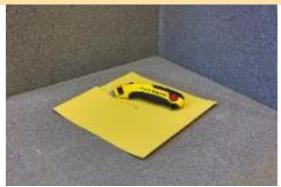
2) Use a hot air gun to shape the membrane properly and adhere the piece onto the concrete using SikaProof® Adhesive-11. Fit the membrane into the edge.
