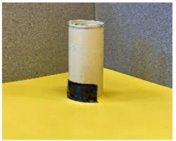
5) Finally adhere a piece of SikaProof® ExTape-150 around the pipe.
