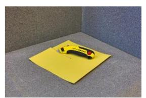
2) Fit the the first single piece of the membrane into the corner, as shown on the picture. Use a hot-air gun to shape the membrane properly.
