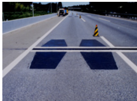
Repairing of cracks and ruts in flooring substrates
