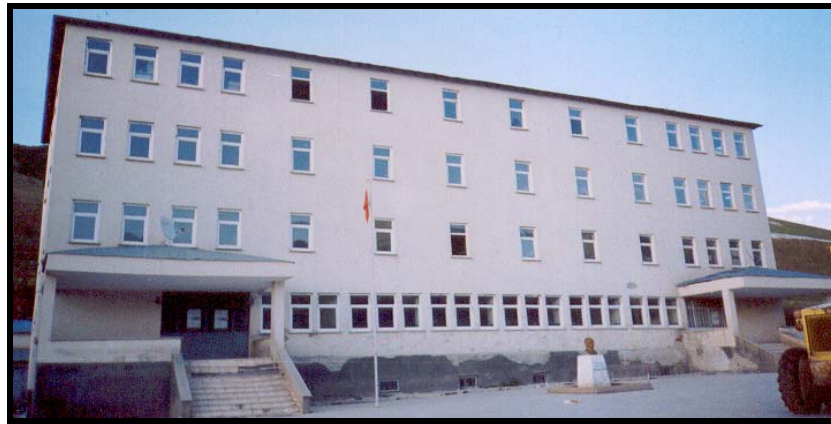
Figure 5.1 Front View of the School Building
