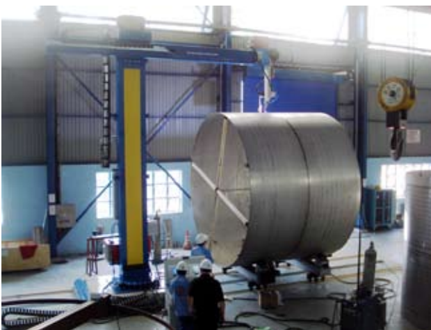
Circumferential welding at tanks with diameter 5.000mm
