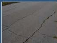
Block cracking typical of CTB.
